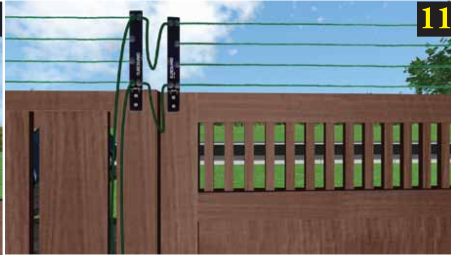
Figure 11 Closeup view of hinged side of gate. A pair of connecting cables joins the fence to the gate. A longer pair of cables are taken down to ground level, across the pathway inside polythene pipe and up the fence on the other side of the gate to continue the barrier. Make sure to tie these cables away from the gate hinge so they cannot be pinched when the gate closes. Bend the poly-pipe into an upside down U so no water enters the pipe.
