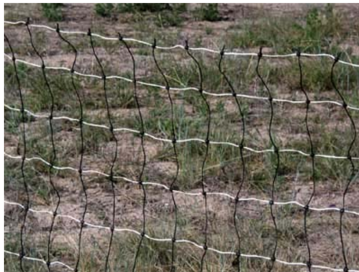
Figure 3b —Unless this fence is kept tight, the flexible vertical strands may allow hot wires to sag, shorting out the fence.
